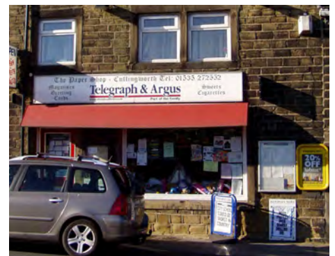
Inappropriate shopfront and clutter at Halifax Road.
