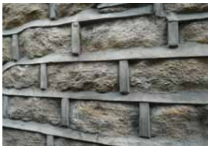
Right: The painting and/or rendering of houses has damaged the character of several buildings within the conservation area. Above: Strap or weatherstruck pointing is not traditional and can harm the look of buildings.
