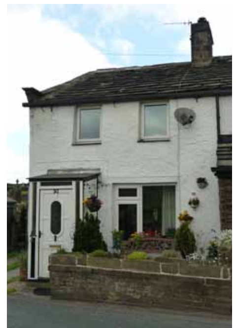
Right: The painting and/or rendering of houses has damaged the character of several buildings within the conservation area. Above: Strap or weatherstruck pointing is not traditional and can harm the look of buildings.
