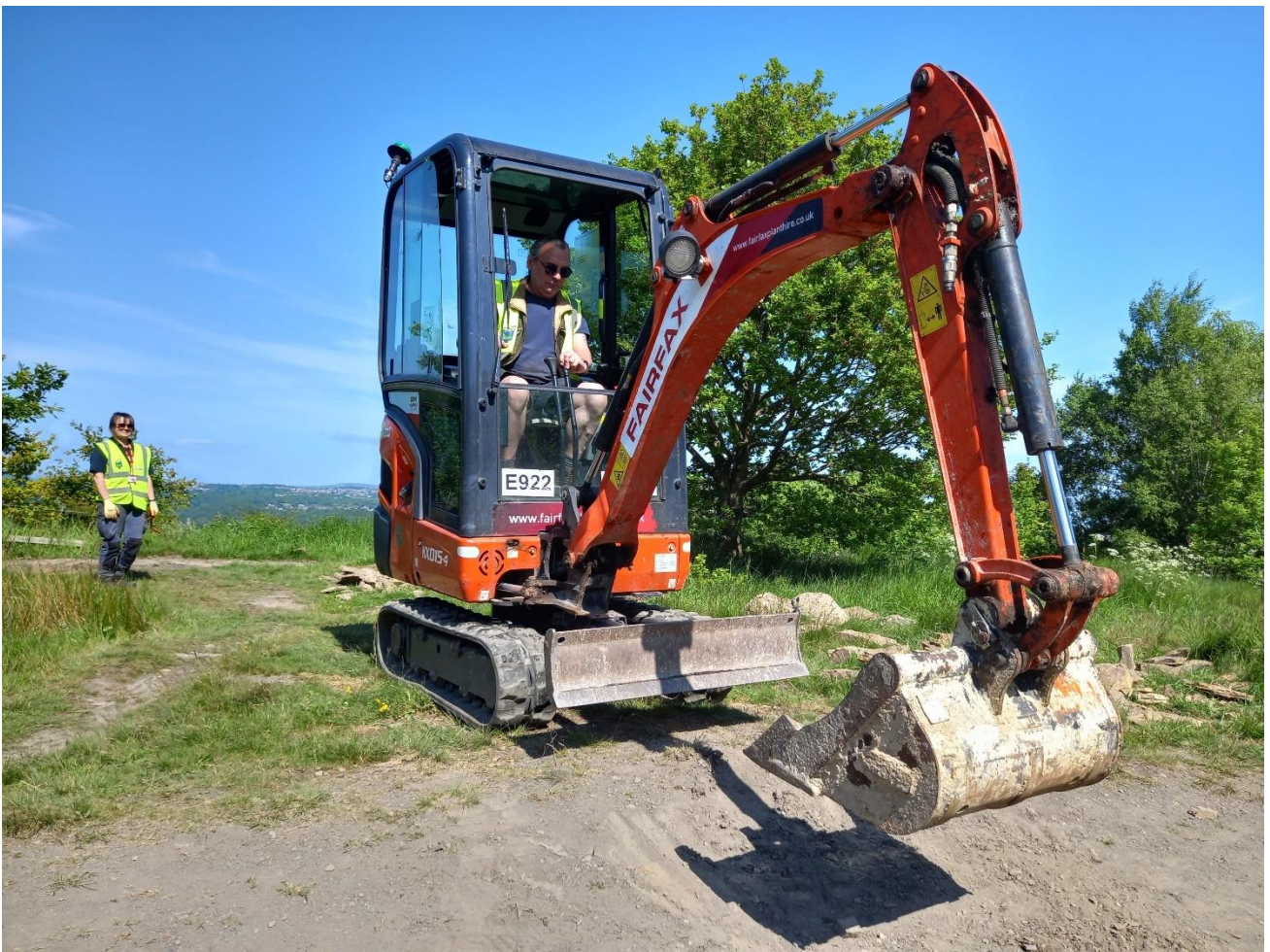
Image: Wrose Quarry Remediation Work
