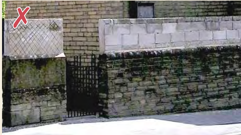
Figure 50: Poor quality and unacceptable addition to stone wall
