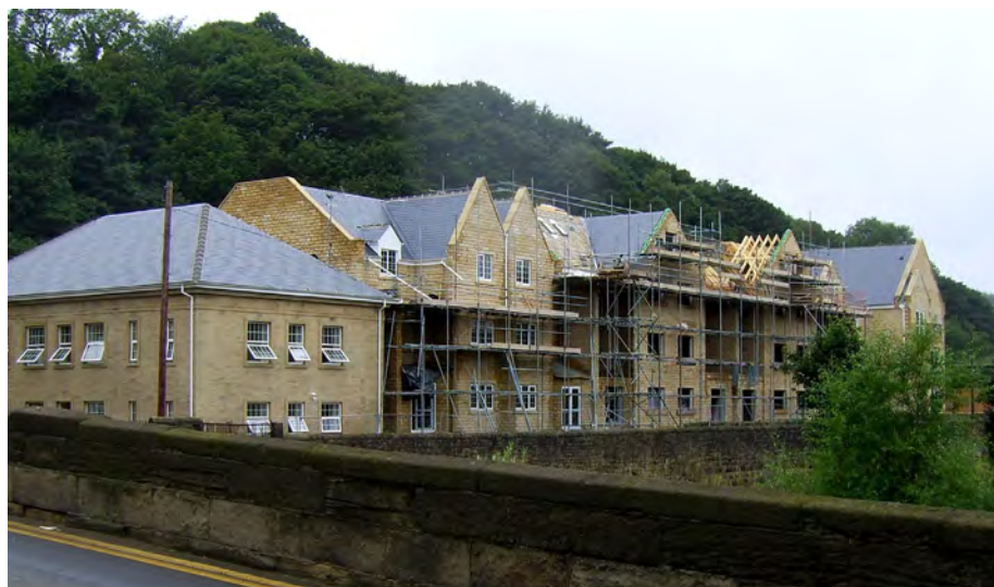
Development in progress alongside the River Aire.
