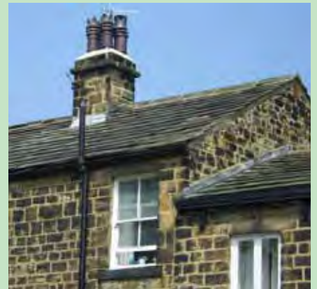
Traditional height chimney and sash detail
