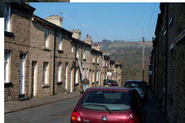
From SP13.5 the caravan site below Baildon Moor is just visible above the rooftops of the western side of Herbert Street.
