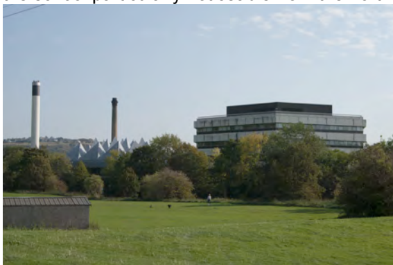
Inland Revenue Building
