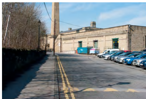
Salts Mill car park and loading bays
