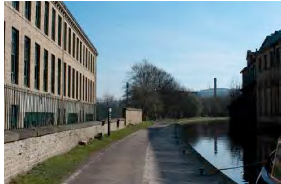
View 7.2 looking east along the Leeds & Liverpool Canal
