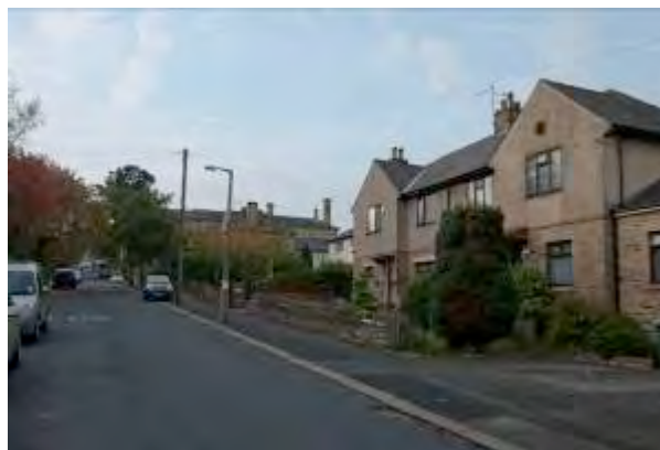
Zone H includes a mixture of post-war housing and school buildings
