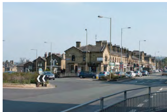
View 29 Bingley Road looking north-east to Saltaire needs revaluation
