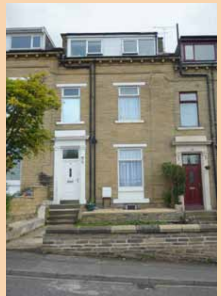
Unsympathetic box dormer windows
