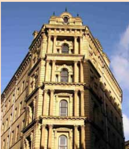
63 Vicar Lane - Little Germany conservation area.
