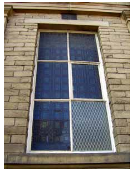
Above: Neglected windows with inappropriate window pane.
