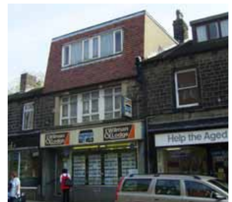
Inappropriate shopfront and dormer window on 70-72 Kirkgate
