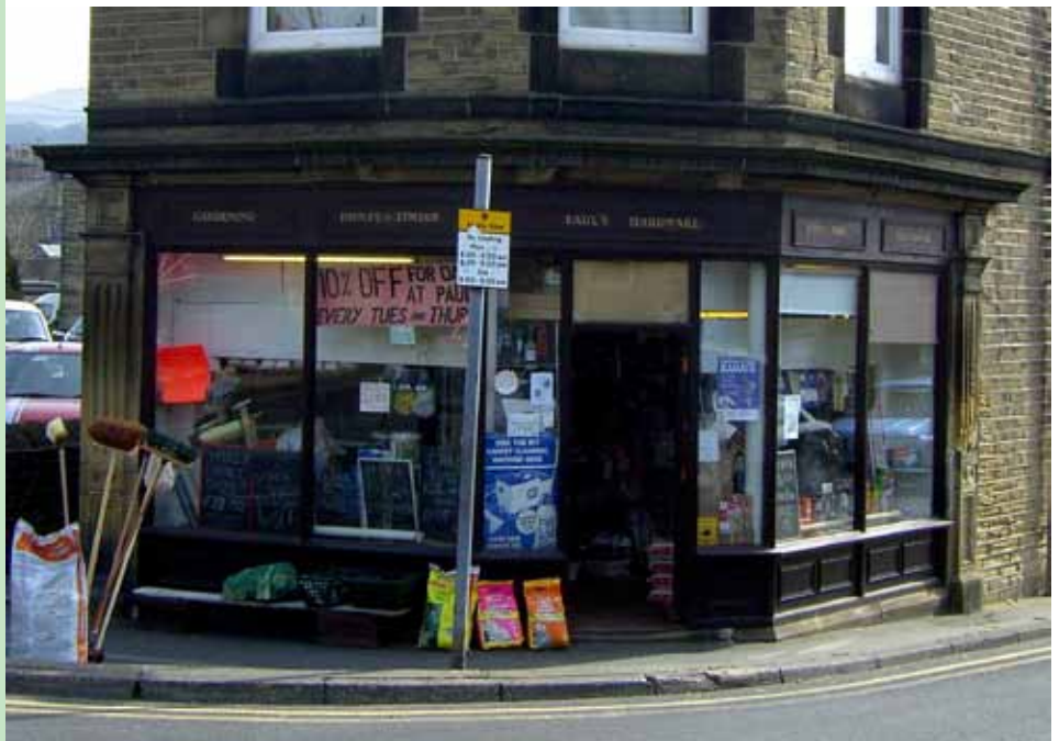
Well detailed traditional shopfront at 26 Briggate
