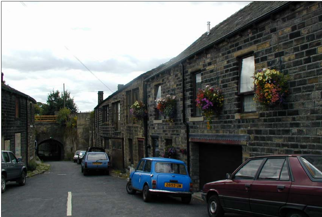
View down Hainsworth Road to the Aqueduct (Grade II) – an attractive street, although part of it is in a semi-derelict state. This is a traditionally industrial part of the settlement: a forge has been on the site of one of these buildings for over five hundred years.
