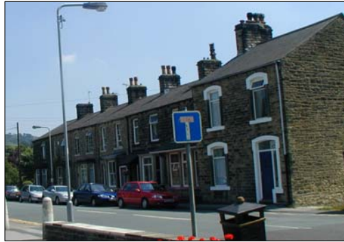
Terrace buildings of Wesley Place (unlisted) – they are typical of the area being constructed of local stone with slate roofs.
