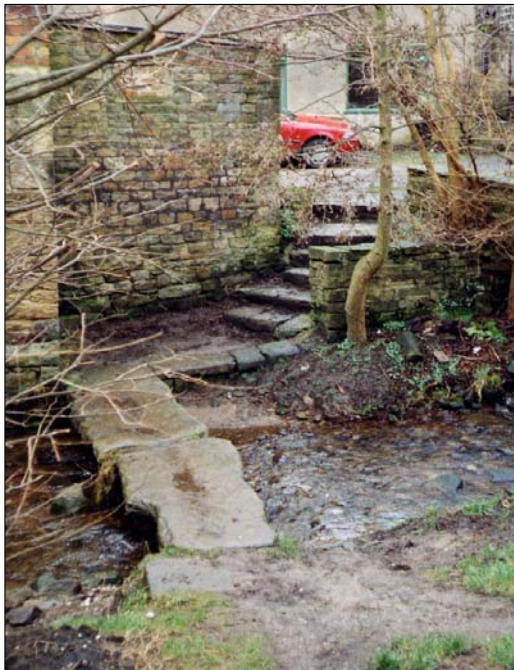
Clapper Bridge – historic bridge crossing the beck.
