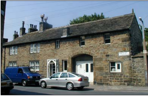
27 North Street (unlisted) – a former laithe house, with characteristic wagon entrance and a stone slate roof.
