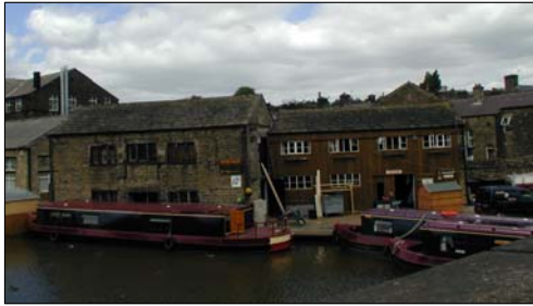
Pennine Boats warehouse (Grade II)
