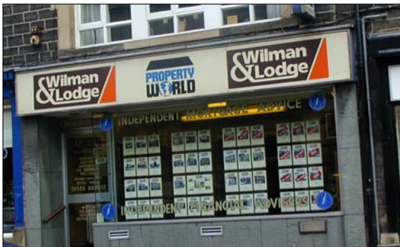
Example of a poorly detailed shop front on Kirkgate, the materials, scale and detail of which is not complementary to the building on which it is situated or the character of the street.
