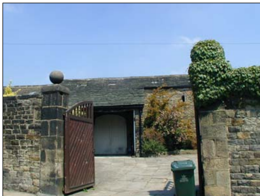
Barn associated with Old Hall Farm (Grade II) – the quality of this area is outstanding.
