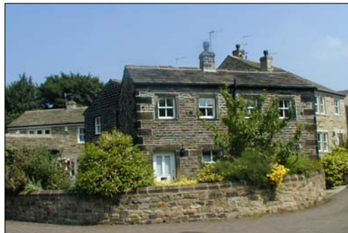
Pear Tree Court – integrating Grade II listed buildings with modern development.
