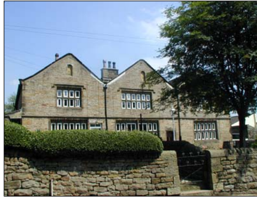
Old Hall (Grade II) – the finest vernacular structure of the settlement.
