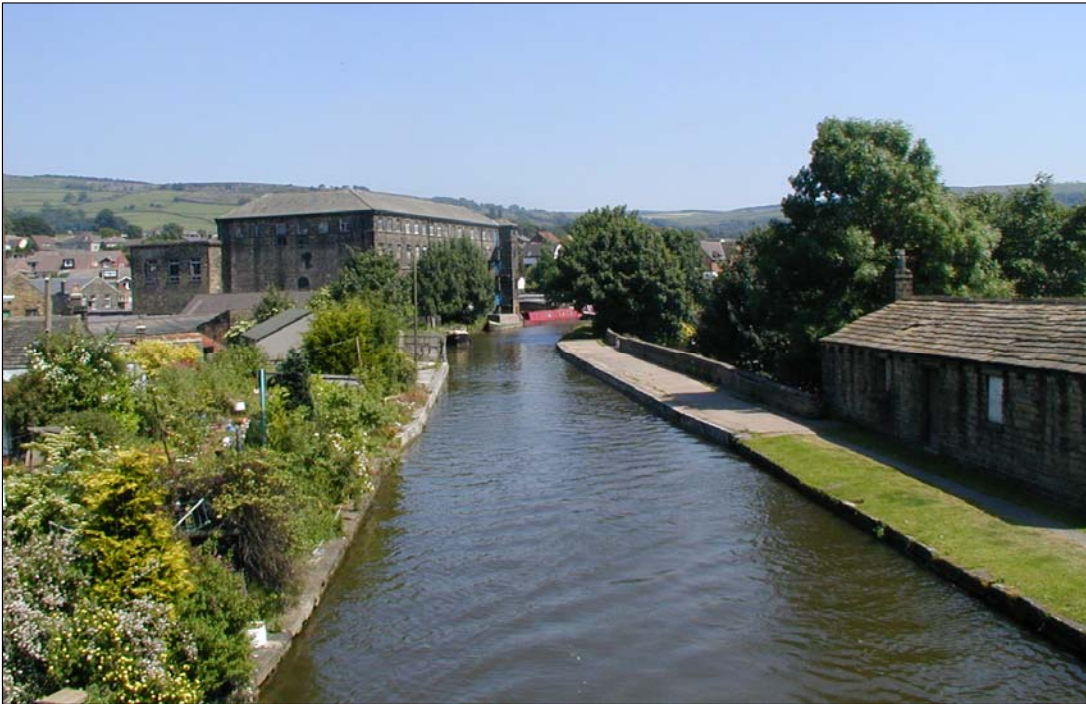
View eastward down the canal to Waterloo Mill
