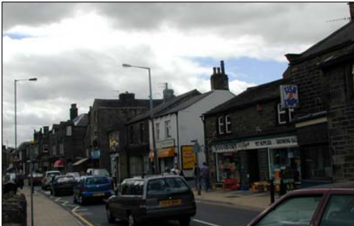
Kirkgate – some of the problems of poor quality signage and shop fronts, street sign clutter and loss of original detail is evident.
