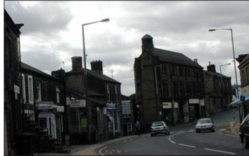
The Co-operative Society building (unlisted) – unusual in design and situated at a prominent terminal point of Kirkgate
