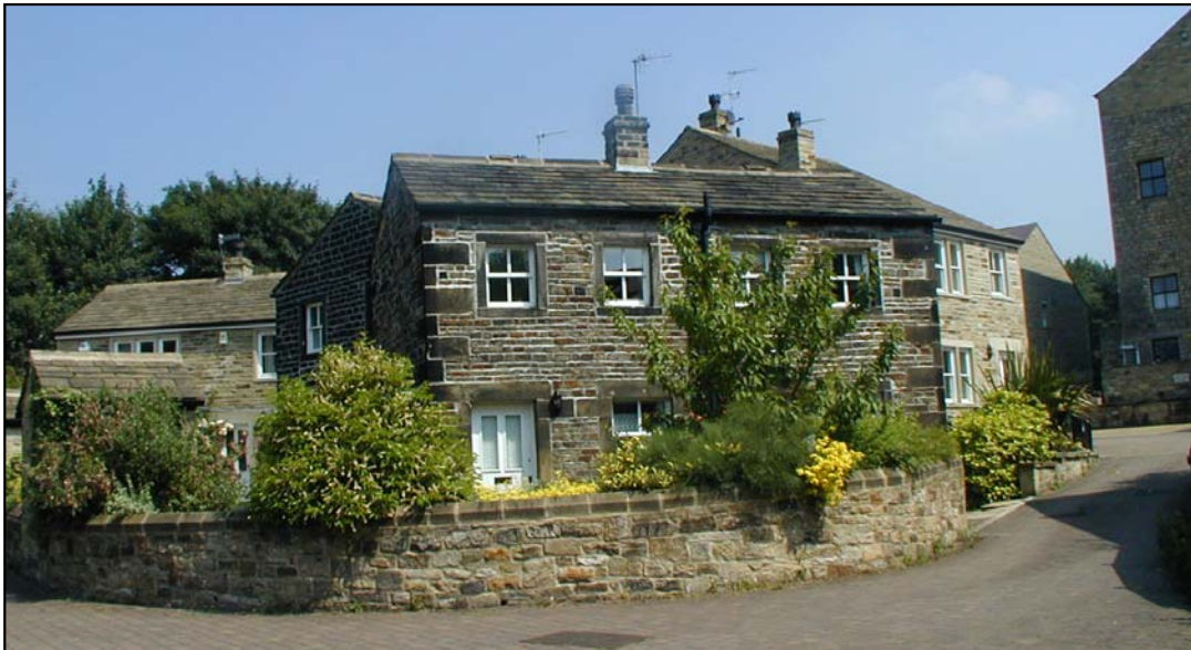
Good quality new development within the conservation area, which is clearly modern, yet integrates well with the adjacent listed buildings
