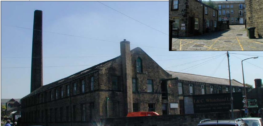
Waterloo Mill – The only Grade II* building in the conservation area and Airedale Mews (unlisted).
