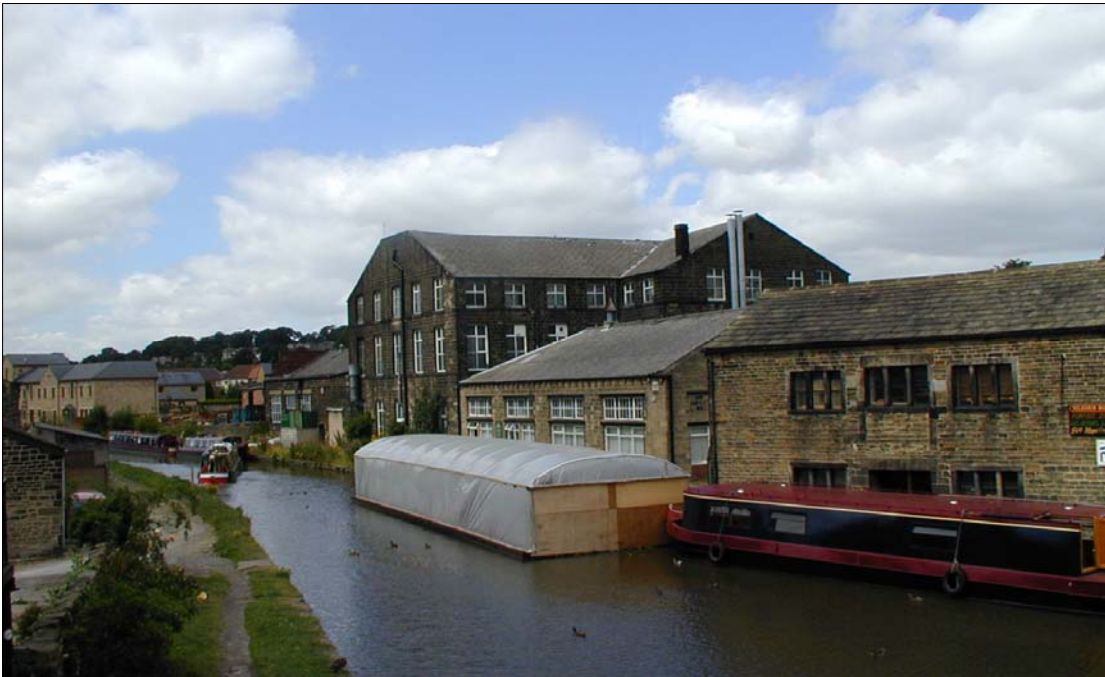
View westward along the canal
