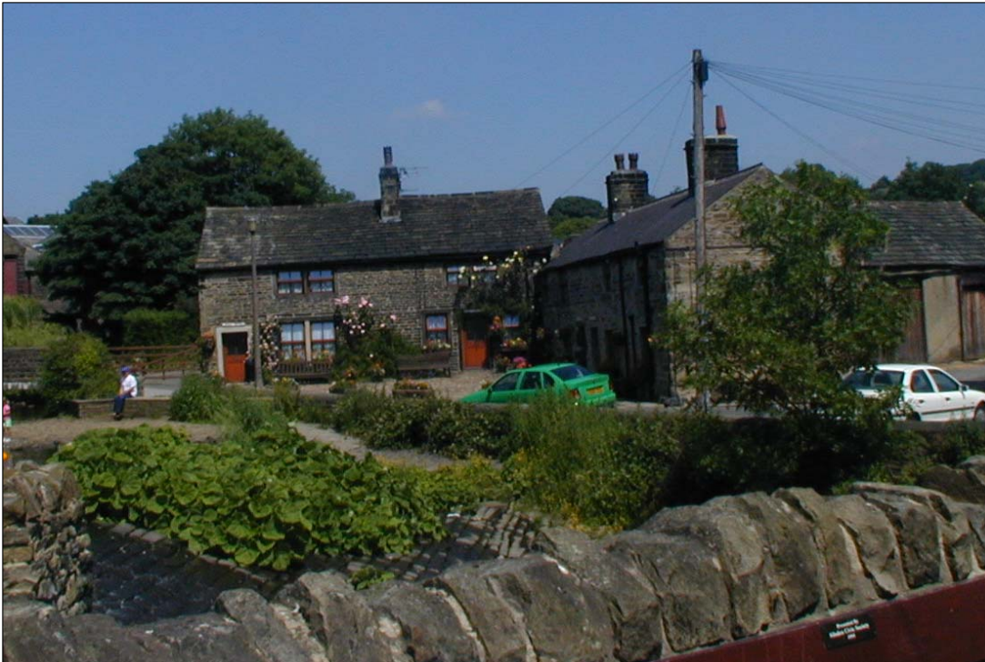
Prominent cottages to the north of St. John's Street (unlisted) – constructed of local sandstone, with stone slate roofs.
