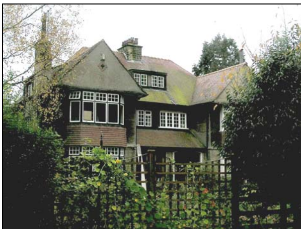
Nos. 9 (North Hill) and 11 (Myddleton Croft) Clifford Avenue.
