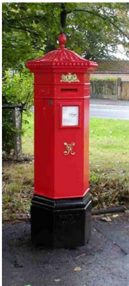
The pillar box on the corner of Middleton Road and Denton Road is a Grade II listed structure. This box is actually a reconstruction of the original box, which was destroyed recently after being hit by a vehicle. The townscape value of structures such as this, which is a particularly rare example of a hexagonal pillar box is high and presumption will always be given in favour of their retention.
