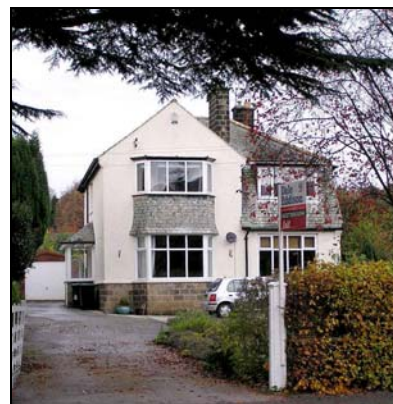
No. 42 Denton Road was built contemporarily with the red roofed houses that line the north side of the road but has a grey slate roof instead.
