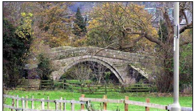
Ilkley Bridge is the historic link between Ilkley and Middleton. The River Wharfe plays an important role in the setting of Middleton.
