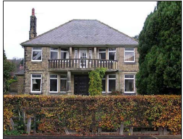
No. 40 Denton Road incorporates some interesting design features, such as the large semi-circular stone balcony to the front elevation.
