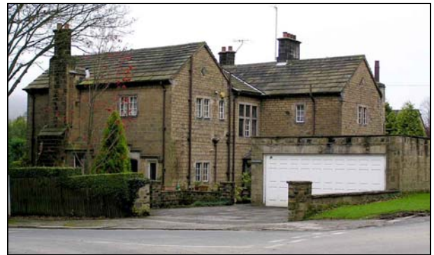
No. 25 Middleton Avenue occupies a prominent plot on the corner of Curly Hill and Middleton Avenue.
