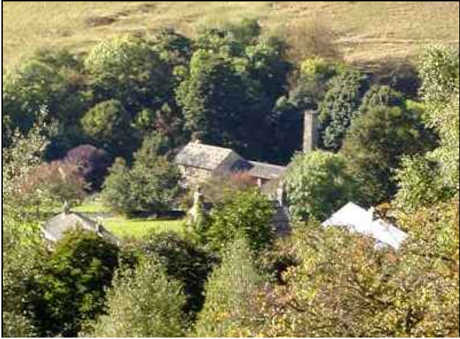
Holroyd Mill and its setting are important unique components of the village's historic fabric which the conservation area has been extended to include
