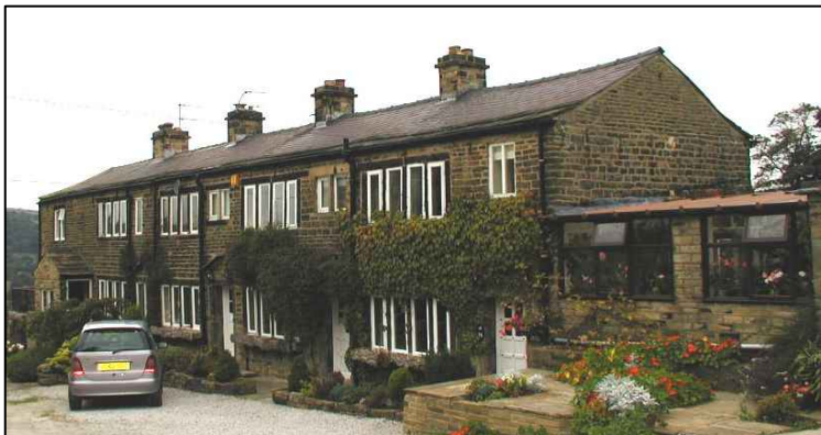
12-20 Victoria Street are the oldest industrial houses in the village, dating from around 1800, and are Listed Grade II. Note the unsympathetic extension to the right.
