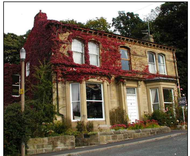
Thornfield House (key unlisted building) retains much of its original character on this elevation which was built in the 1870s.
