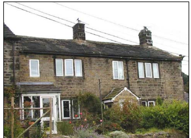
2-4 High Fold (unlisted) is a pair of cottages with the chimneys, quoins, date stone and decorative kneelers of an earlier building.
