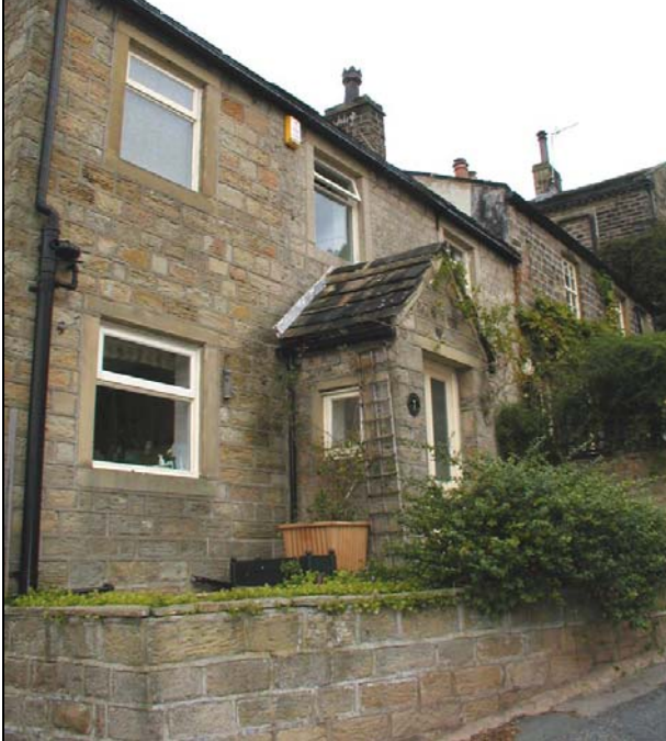
37 Micklethwaite Lane is a two-bay cottage which has been extended with a sympathetically proportioned and detailed single bay extension to the left which uses a good match of stone.
