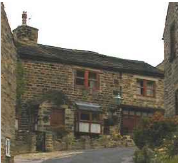
33-35 Micklethwaite Lane is a cottage from around 1800 which has been thoughtfully extended to the right with a good match of details, materials and proportions.
