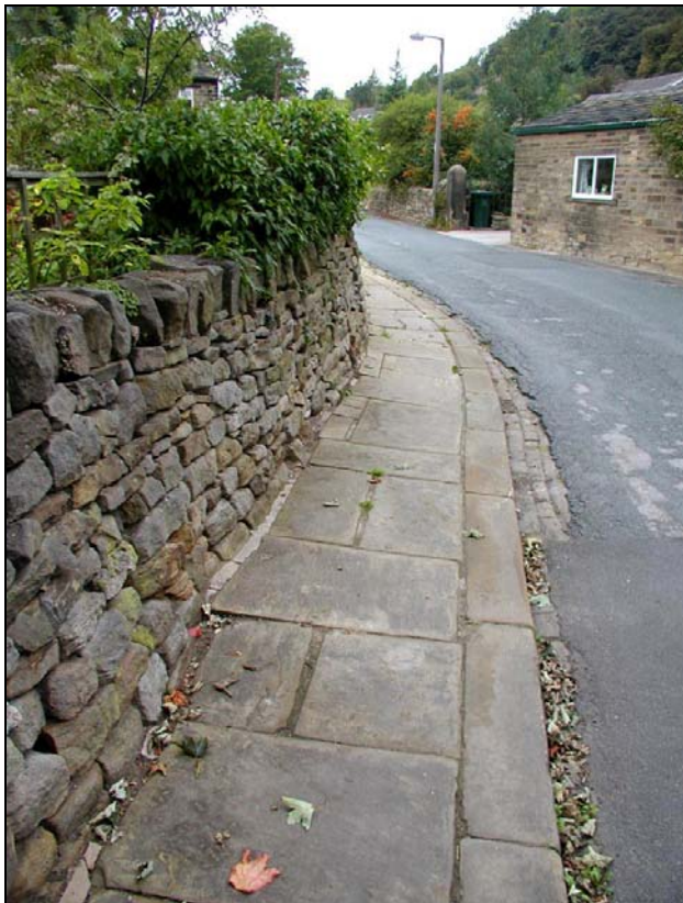
Stone walls, and where they exist, flagged and setted surfaces enhance the appearance of Micklethwaite Lane and add to its historic character.
