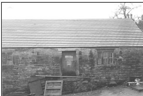
This historic photograph shows what the Grade II Listed Micklethwaite Malthouse looked like when it had a modern tile roof. The building is now sympathetically roofed in stone.
