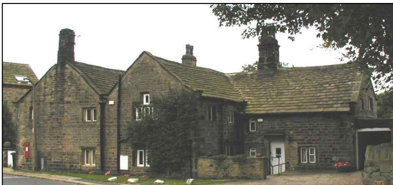
21-23 Micklethwaite Lane (Micklethwaite Grange). The layout of the Grange is unusual with two gable-fronted blocks with a double span roof to the left.
