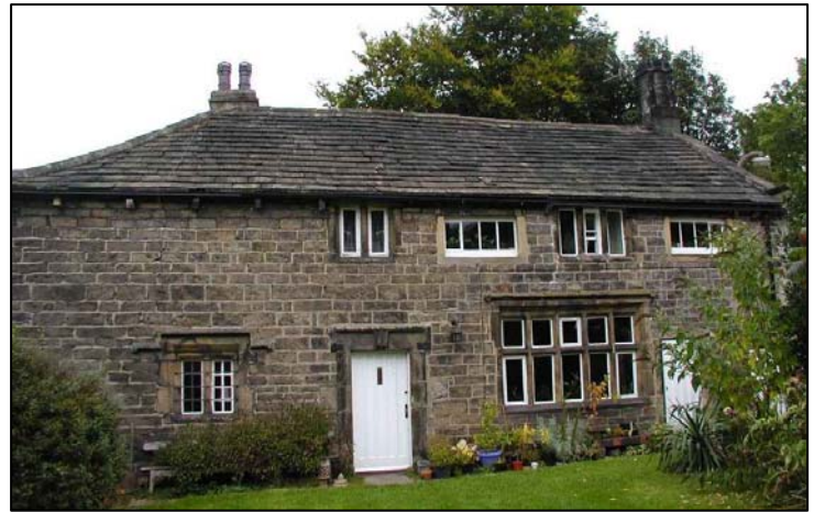
21 Micklethwaite Lane (Micklethwaite Grange) is dated 1695. This Grade II Listed building retains many of its original details. The first floor windows lacking mullions were inserted during the mid-20 th century.
