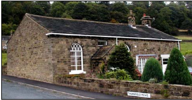
Overcroft (unlisted) was built as a Methodist Chapel in 1854. The round-headed windows with astragal uppers are an important original detail.
