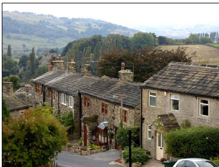
The two two-storey, single bay extensions in this picture (one behind the lamp post, another to the right of it) show how a good match of materials and a careful consideration of traditional details, building techniques and the wider character of the street can lead to new development which is in keeping with the conservation area.
