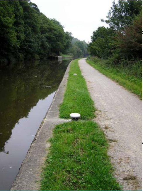
The concrete canal bank at the edge of Riddlesden is out of place in a rural scene such as this.
