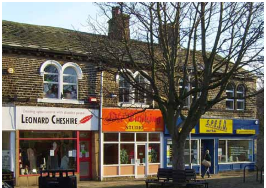
Altered and modern shopfronts, The Green
