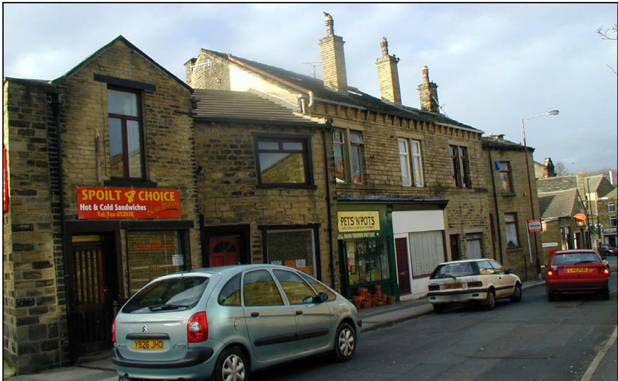
Stepped frontages of the individually designed buildings of Bradford Road – fronting directly onto the street, as is typical of the conservation area, illustrative of the haphazard feel of the built fabric of The Green.
