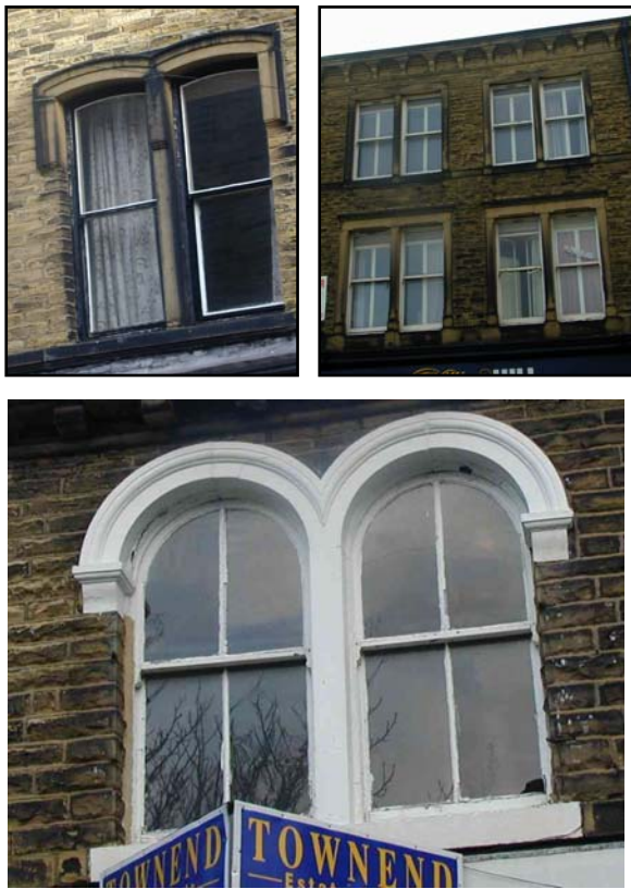
Examples of different mid-late nineteenth century window surrounds with good quality timber sash windows.
