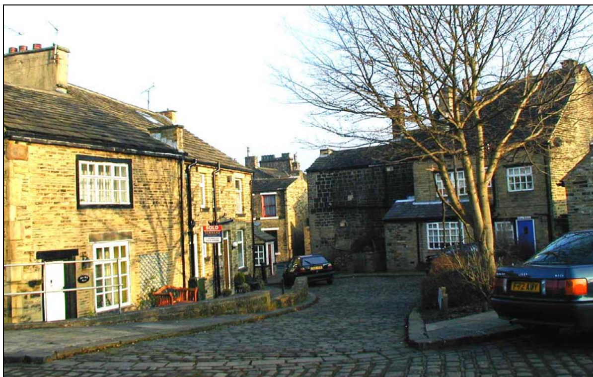
Eighteenth century cottages clustered around North Fold – reminiscent of a bygone age when Idle was a rural village. Unfortunately, over time the original window detailing has been lost as replacement windows are made of different materials such as uPVC and feature different openings such as casement instead of sash, while the windows themselves are no longer recessed.
