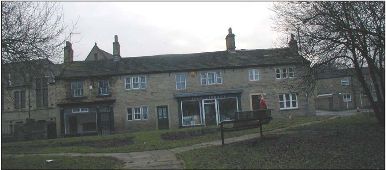
18 – 22 Albion Road (Grade II) – early nineteenth century examples of vernacular two-storey stone cottages with stone slate roofs, plain stone door and window surrounds and mullioned windows that retain their original glazing pattern
