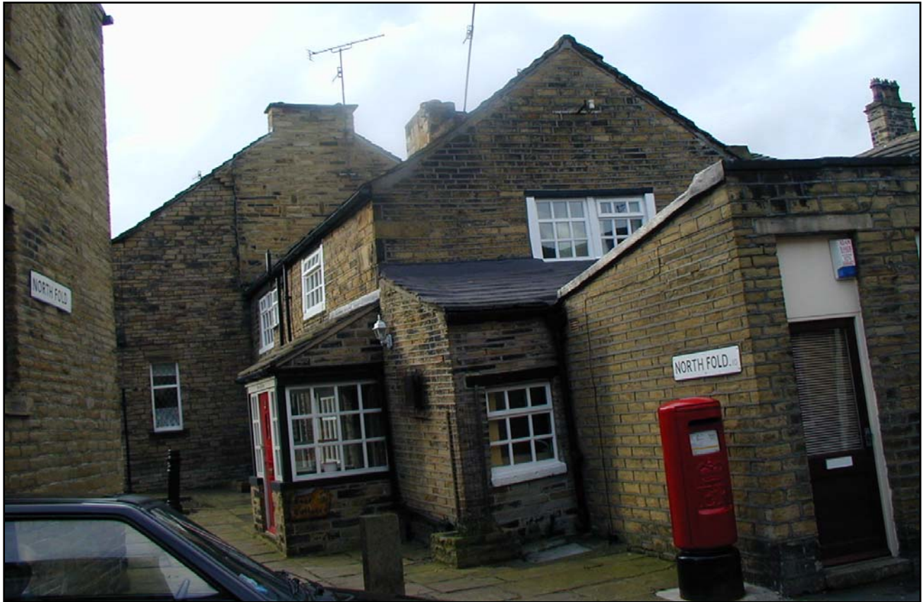
View into North Fold from Bradford Road, with its collection of small, irregularly orientated cottages creating an enclosed space with an intricate building form.
