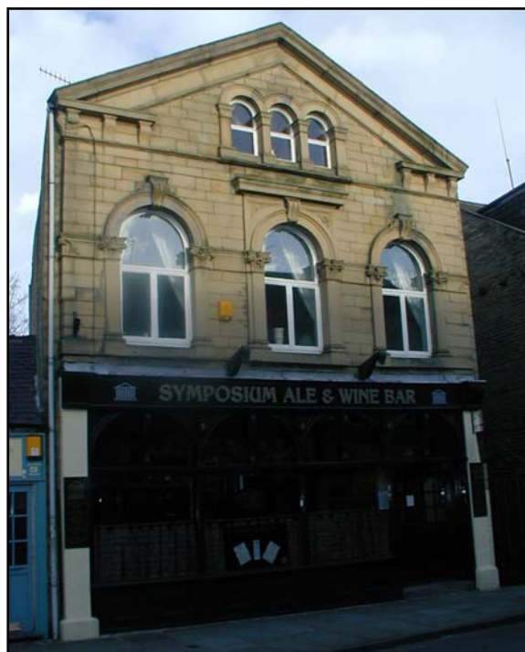
7 Albion Road – two and a half storey Italianate style structure.
