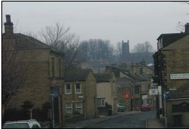
Entrance into The Green Conservation Area from Bradford Road – due to its elevated position the tower of Holy Trinity Church dominates the skyline.
