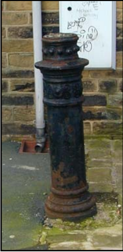
This iron bollard at entrance to Southcote Place from Bradford Road might well have originally been the base of a lighting column.
