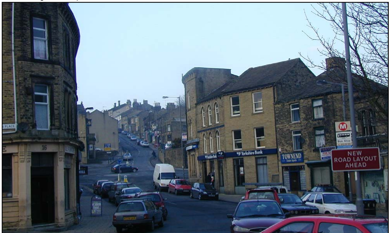
Visual link between The Green Conservation Area and Idle Conservation Area – important to an understanding of the development of the settlement. The clutter created by a surfeit of signs mars the area's historic appearance.
