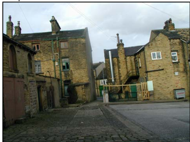
Rear of 26 – 28 The Green and 2-4 Albion Road from Southcote Place – the alley between the two allow permeability through the site.
