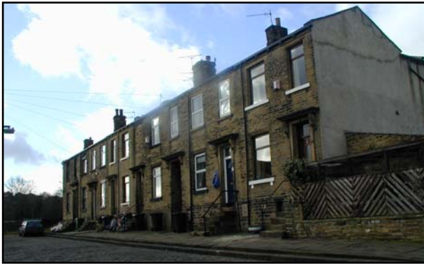
Victorian Terraces on Walter Lane – constructed of local stone with stone slate roofs, stone chimneys and more ornate door surrounds
