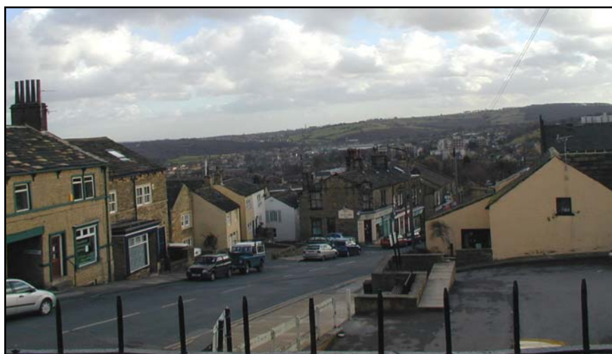
View southwards from Town Gate – the topography gives Idle a hilltown character. Visual connections with surrounding moorland are opened up and the roofscape of High Street becomes a particularly important feature of the village.
