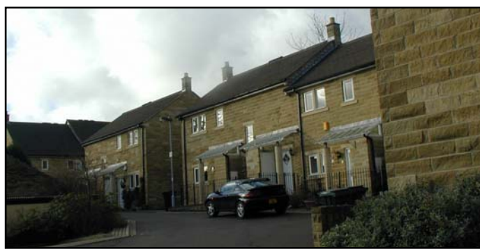
Example of modern an interesting housing development that is sensitive to the local vernacular style of architecture that is reflected in the well chosen stone and cut mullioned windows. Pastiche is avoided by the imaginative use of modern-style glazed porches on stone columns and projecting bays, topped by timber windows under the eaves of the slate roofs that have varying rooflines. The chimneys reflect the traditional detail of the area.
