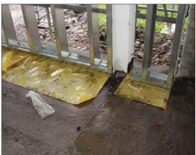
Figure A4.80 Column left unsealed (courtesy PAGeotechnical Ltd)
