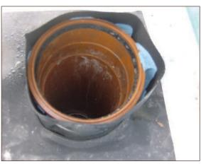
ure A4.74 Gap between OD of service pipe and ID of top hat to large: cannot be compressed enough to form seal, even with the application of additional tape (courtesy Smith Grant)
