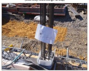
Figure A4.9 On site schematics to aid construction workers build the gas protection system (courtesy Alderburgh Group)
