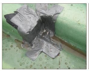
Figure A4.69 Attempt at corner detailing using nonproprietary duct tape (courtesy Smith Grant)
