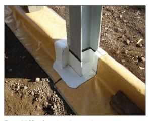
Figure A4.23 Complex column seal (courtesy PAGeotechnical Ltd)
