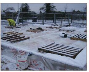
Figure A4.84 Taped joints are difficult to construct in adverse weather. Also difficult to inspect if covered with snow (courtesy Smith Grant)
