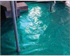
Figure A4.52 Gas membrane cut by scaffolders and bricklayers after installation (courtesy MEC Environmental Ltd)
