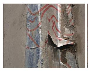
Figure A4.55 Gas membrane at stepped junction of slab to integral garage, appears to be susceptible to tearing when screed is poured. Screed may also weigh down on gas membrane if fitted too tight (courtesy NHBC)
