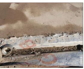
Figure A4.56 Gas membrane at edge of concrete screed.
