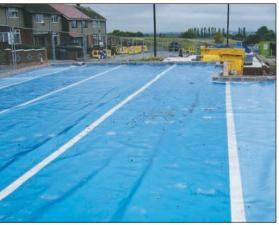
Some stones could penetrate gas membrane if sufficient force is applied (courtesy Smith Grant)
