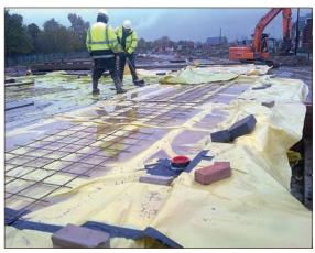
Figure A4.67 Traffic over mesh resulted in several punctures, in addition most joints were found to be poorly constructed. Taped joints are difficult to construct in adverse weather (courtesy Smith Grant)
