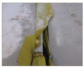
Figure A4.79 Gas membrane not continuous over internal Figure A4.80 wall. It had been deliberately cut open for unknown purpose (courtesy Smith Grant)
