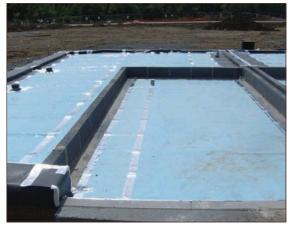
Figure A4.11 Gas membrane continued through cavity wall and above air bricks (courtesy Hydrock)
