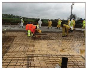
Figure A4.57 Unprotected gas membrane damaged by heavy traffic (courtesy MEC Environmental Ltd)
