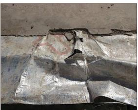
Gas membrane damage/tearing at edge of ground floor slab screed layer where it was left exposed to elements for period of time (courtesy NHBC)
