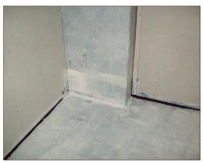
Figure A4.83 Poor quality installation of liquid gas membrane. Liquid gas membranes come in two colours (black and white) allowing coverage of each coat to be easily assessed. Here the gas membrane has been spread too thinly and inconsistently. In addition, it appears to have been applied to a damp surface, causing blistering (courtesy Card Geotechnics Limited)
