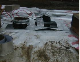
Figure A4.72 Joint between top hat and gas membrane has lifted due to poor fit and attempt to construct in very wet conditions (courtesy Smith Grant)
