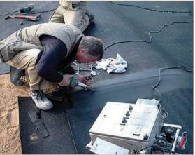
e A4.42 Air pressure testing (courtesy GSE Environmental)
