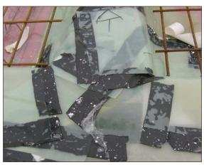
Figure A4.68 A pre-formed corner unit would have been preferable. The installer could not produce sufficient quality despite the amount of tape applied (courtesy Smith Grant)
