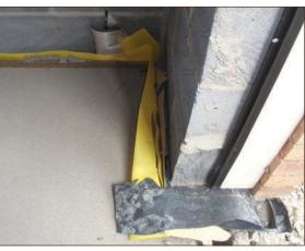
Figure A4.70 Inadequate corner detailing. The use of preformed proprietary products would have avoided such bad practice (courtesy NHBC)
