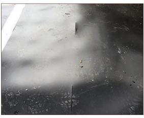
Figure A4.58 Damage caused to gas membrane by follow-on trade who cut/shaped the dry lining board directly on the unprotected installed gas membrane (courtesy NHBC)
