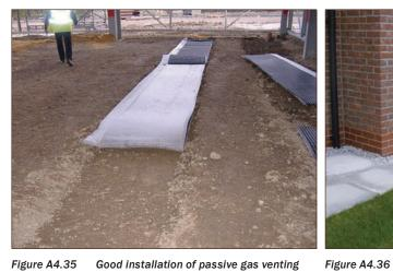
Figure A4.35 Good installation of passive gas venting trenches and 'egg-crate' (courtesy Card Geotechnics Limited)
