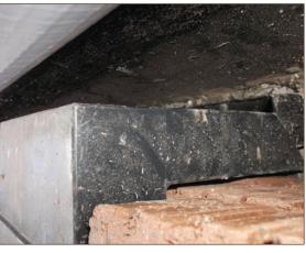
Figure A4.88 Ventilator becoming detached to fit to external block work. This is due to builders requiring increased cavity widths to achieve thermal properties expected by Building Regulations (courtesy NHBC)
