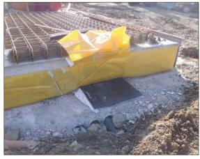
Figure A4.7 Geovent protruding out of the frontage of the unit. Gas membrane along the sides of the slab preventing lateral gas ingress (courtesy Alderburgh Group)
