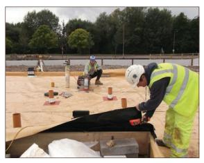
Figure A4.37 Tracer gas testing, whereby gas or smoke is applied under pressure beneath the installed gas membrane and detectors are used to screen for leaks above (courtesy NHBC)
