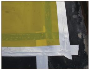
Figure A4.19 Well-constructed joints with gas resistant DPC, lap and double sided butyl joints visible beneath semi-transparent gas membrane, secondary seal with proprietary single sided tape (courtesy Smith Grant)
