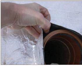
Figure A4.73 No bead of double sided butyl tape provided between interfaces of ID top had and OD service pipe: cannot be compressed enough to form seal (courtesy Smith Grant)
