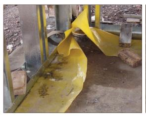
Figure A4.81 No seal to perimeter pipe (courtesy PAGeotechnical Ltd)
