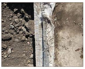
Figure A4.53 Gas membrane left exposed for long period of time, shows significant fraying at cavity edge (courtesy NHBC)
