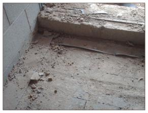
Figure A4.63 Absence of surface preparation prior to laying of gas membrane, debris likely to pierce gas membrane (courtesy Card Geotechnics Limited)
