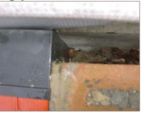
Figure A4.86 Cavity is becoming blocked with detritus.
