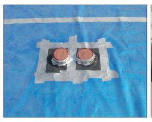
Figure A4.27 Top hats placed around service entries secured with jubilee clip seals. Top hats secured to gas membrane with double sided butyl tape (courtesy Hydrock)
