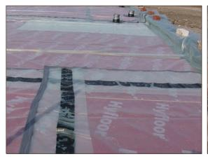
Figure A4.65 Wrinkling of gas membrane over joint has resulted in gaps (only visible due to the use of a transparent gas membrane) and the secondary seal uses ordinary gaffer tape rather than a proprietary product (courtesy Smith Grant)
