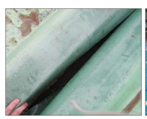
Figure A4.59 Gas membrane slit at the bottom of a cavity Figure A4.60 tray to enable water to drain away (courtesy Smith Grant)
