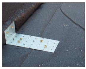
Figure A4.47 Follow-on works purposefully penetrating gas membrane (courtesy Card Geotechnics Limited)
