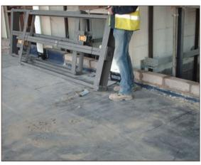
Figure A4.50 Large/heavy/sharp objects being moved over unprotected gas membrane (courtesy Card Geotechnics Limited)
