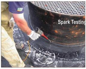
Figure A4.45 Spark testing (courtesy GSE Environmental) Figure A4.46
