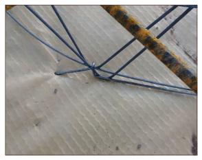
Figure A4.51 Gas membrane torn by reinforcement (courtesy MEC Environmental Ltd)
