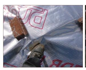
Figure A4.71 No corner detailing leading to stress point on gas membrane (courtesy Smith Grant)
