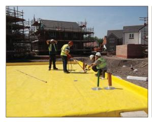
Figure A4.43 Dielectric porosity testing for housing scheme (courtesy NHBC)
