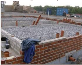
Figure A4.85 Clean single sized stones with no fines acting as venting media, however no ventilation gaps in internal sleeper walls (courtesy Smith Grant)
