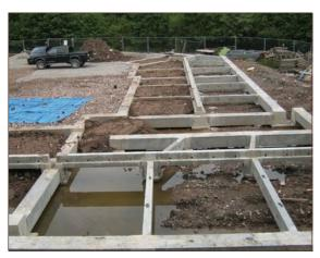
Figure A4.33 Good ventilation in internal sleeper walls, cast into prefabricated beams (courtesy Smith Grant)
