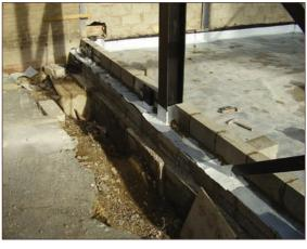
Figure A4.12 Good edge detail across cavity (courtesy PAGeotechnical Ltd)
