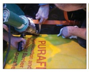
Figure A4.29 Extrusion welding technique (courtesy Industrial Textiles & Plastics Ltd)
