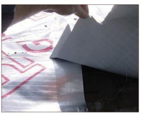
Figure A4.76 No double sided tape used in joints (courtesy Smith Grant)
