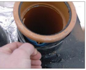
Figure A4.28 Bead of double sided butyl tape provided between interfaces of ID top hat and OD service pipe. When compressed with jubilee clip, forms an effective seal (courtesy Smith Grant)
