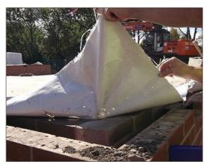
Figure A4.49 Lifted gas membrane at corner position.
