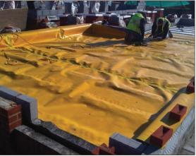
4.18 Gas membrane installed as part of foundation barrier (courtesy Industrial Textiles & Plastics Ltd)
