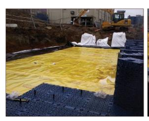
Figure A4.17 Gas membrane installed in attenuation tank (courtesy Industrial Textiles & Plastics Ltd)
