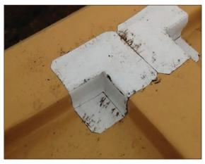
Figure A4.21 Good prefabricated corner detail (courtesy MEC Environmental Ltd)
