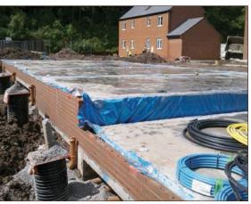
Figure A4.82 Gas membrane used to bridge cavity wall instead of DPC, leaving it exposed to damage by follow-on trades (courtesy Smith Grant)
