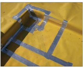
Figure A4.20 A pre-formed corner unit would have been preferable as fewer joints would have been formed, however the installer has achieved a good level of workmanship in this corner detail (courtesy Smith Grant)
