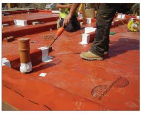
Figure A4.39 Scanning for leaks (courtesy PAGeotechnical Ltd)
