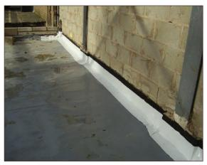
Figure A4.14 Good perimeter seal (courtesy PAGeotechnical Ltd)
