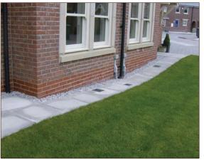
Raised air bricks are preferable due to the reduced potential for blockade but the vent trench specified is provided with clean single sized stone (courtesy Smith Grant)
