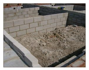
Figure A4.89 No ventilation in internal sleeper wall (courtesy Smith Grant)
