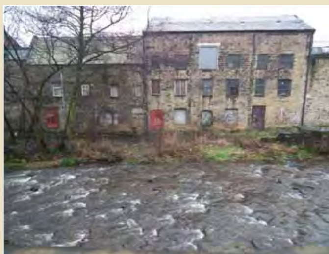
Buildings in poor condition on Beck Street
