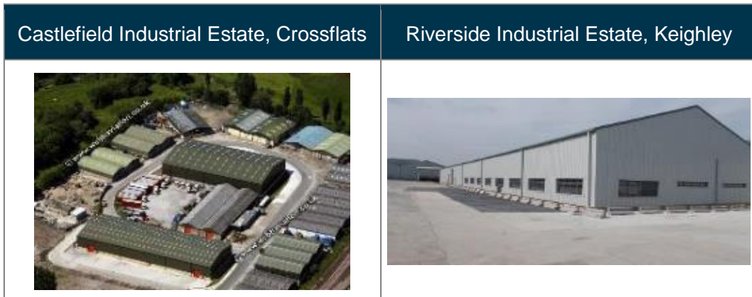
Figure 4.19 – Examples of industrial space in Airedale
