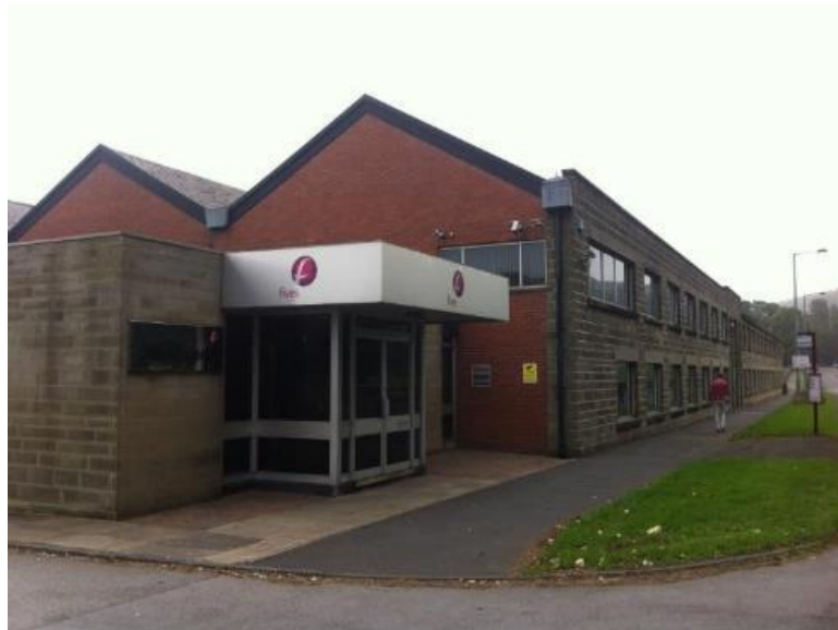
Eastburn Works, Skipton Road, Eastburn
