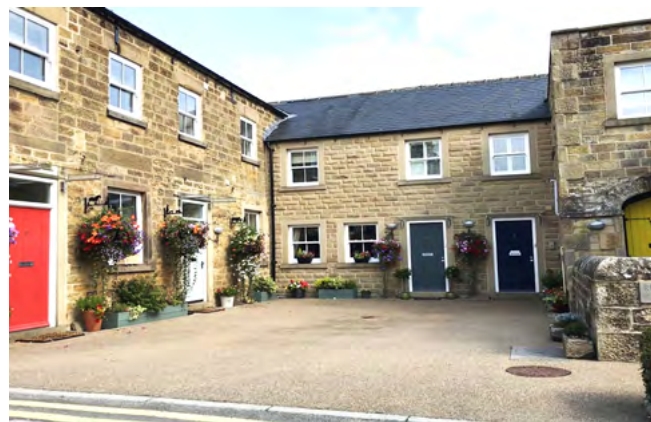
Individual painted doors in courtyard
