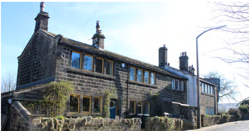
13 & 17 Hebden Bridge Road
